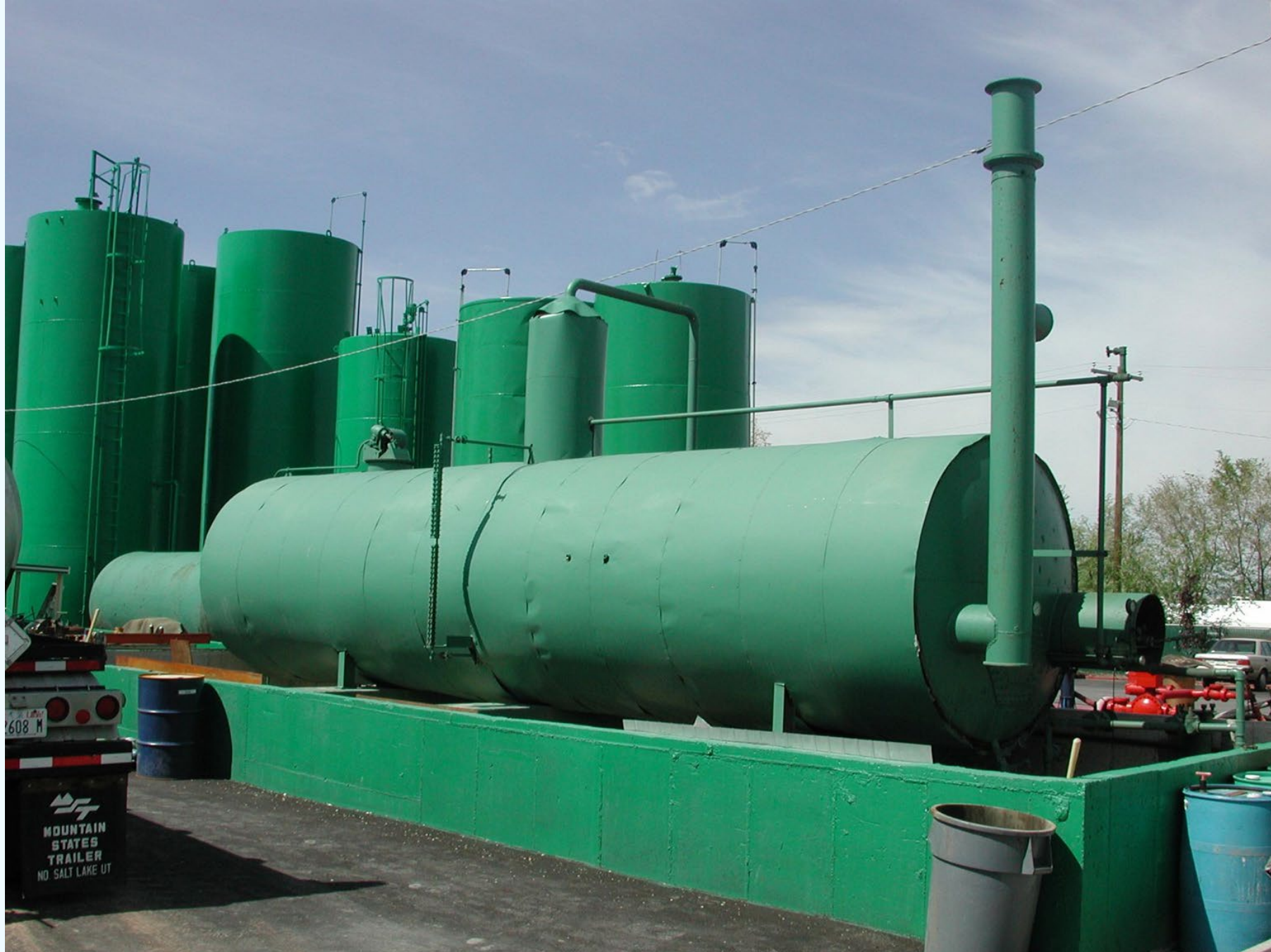
One of the former local processor facilities.
